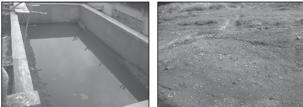
Fig. 3. Recharge Shaft(Left) and its rainfall catchment area.
