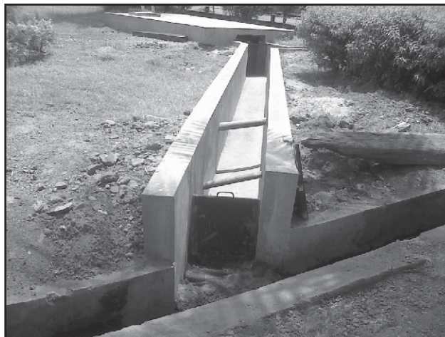
Fig. 2. Final Photo of Recharge Pit with water regulators for existing drain
